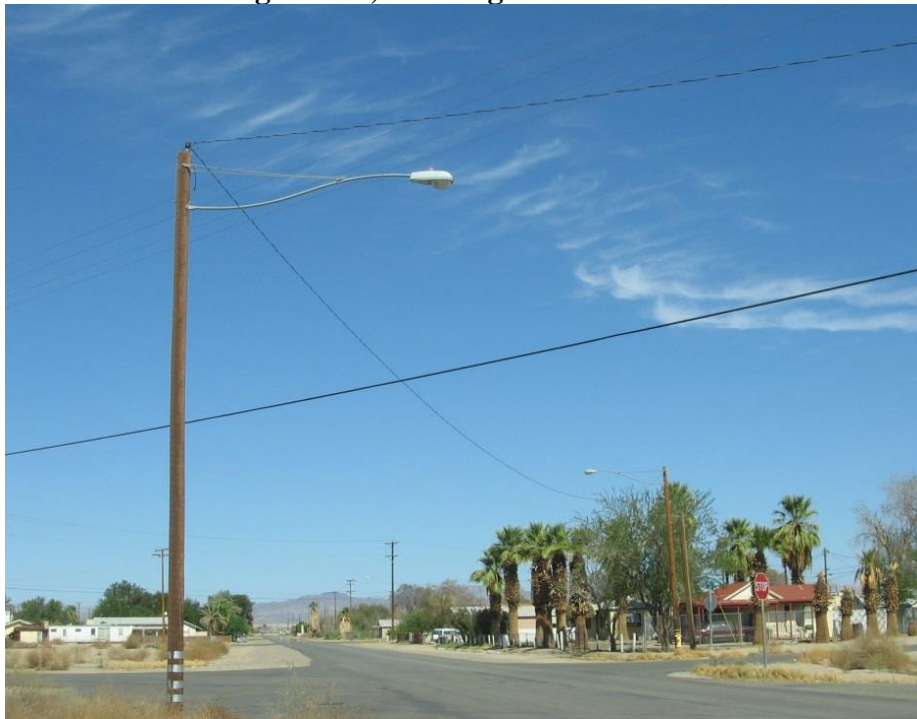
Existing streetlight located along Main Street
